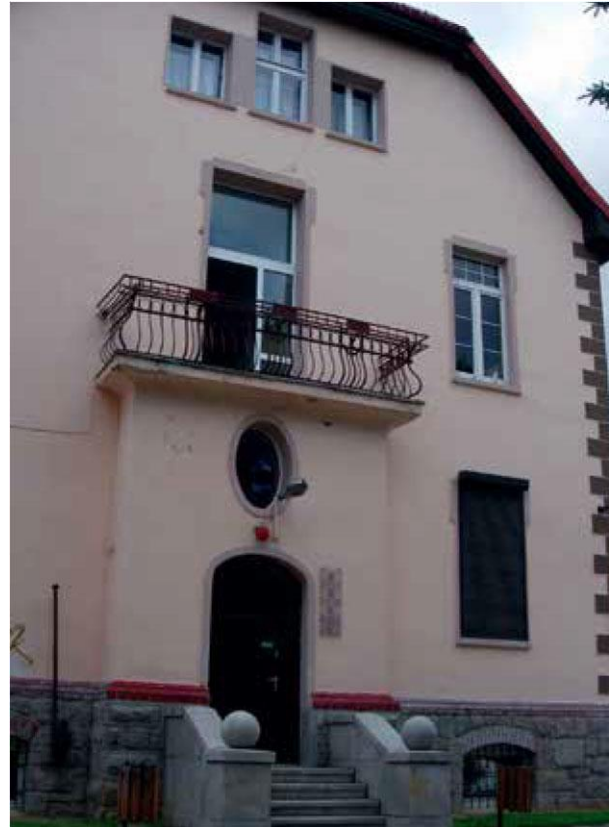
Figure 4. Main entrance to former City Hospital in Sobótka from Świętego Jakuba Street (formerly 28 Armii Czerwonej Street), Sobótka, 2015 (photo by Z. Kopociński)
